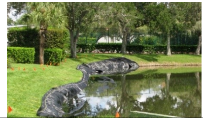
Tubing to Stabilize the Bank
